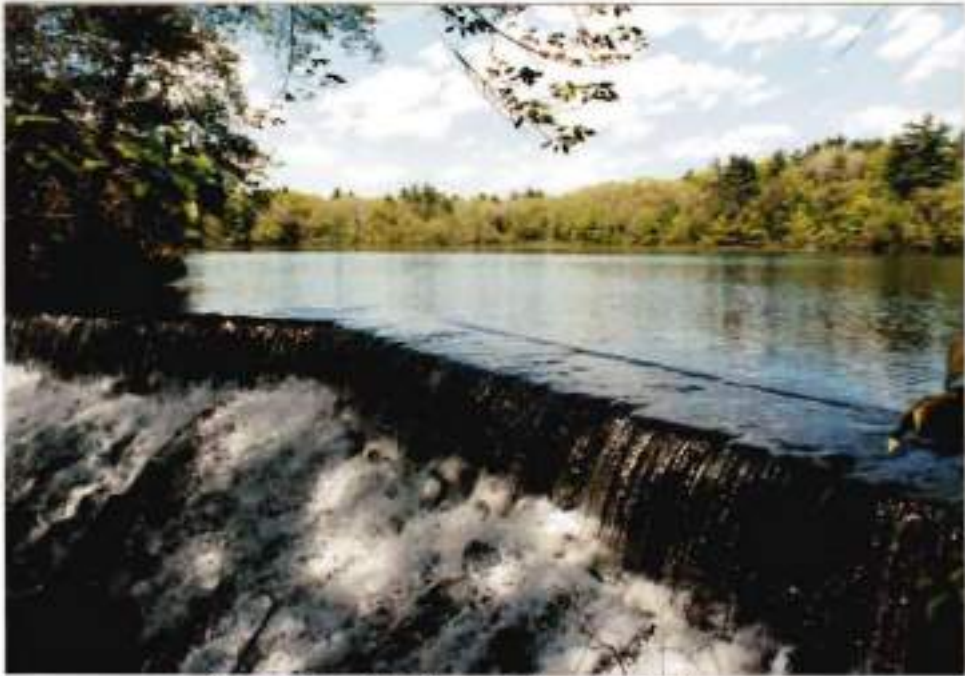
Looking NE from the spillway on the dam.
